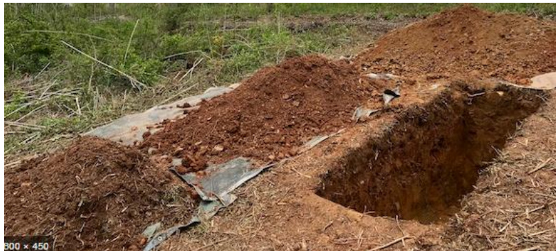
Fig 2.1. Removing the topsoil
